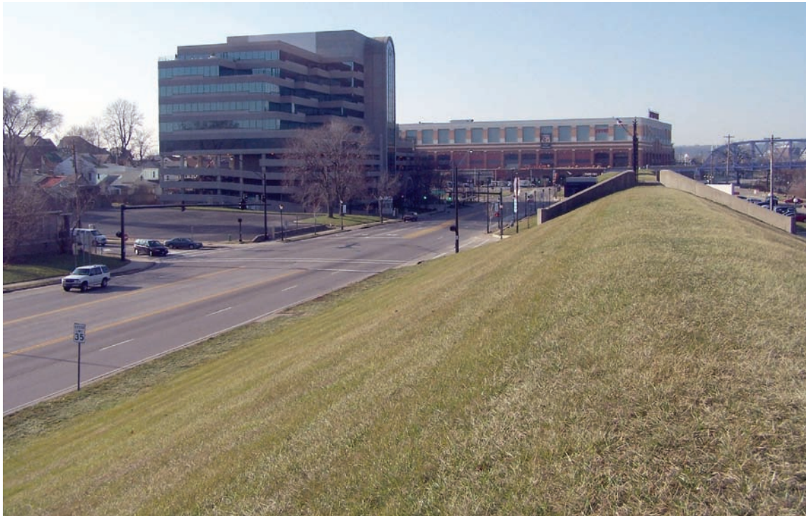
The levee in Newport in Campbell County, looking north toward the Newport Aquarium (center). Newport has an excellent system of levees to protect the city from flooding by the Ohio River. Photo by Richard Smath, Kentucky Geological Survey.
